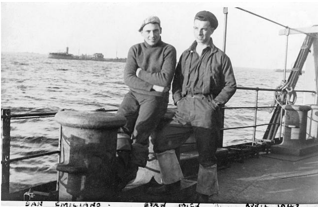
Image 9 is an enlargement of Image 8 to highlight the Degaussing cables fitted to San Emiliano . Degaussing reduced the risk of ships being detected by magnetic mines and was initially fitted externally as shown here. The thick cables carrying the degaussing current are to be seen strapped to the diagonal metal trough.
